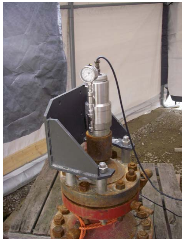
Figure 3 MP55 Well Head Completion – DGR-2
